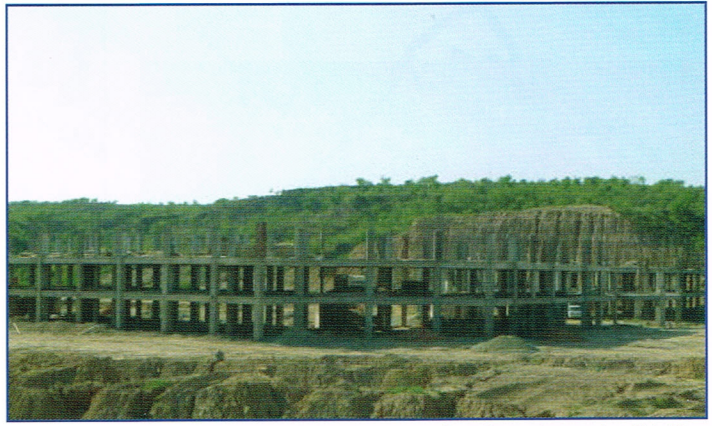
KORT Educational Complex work started on Third floor
