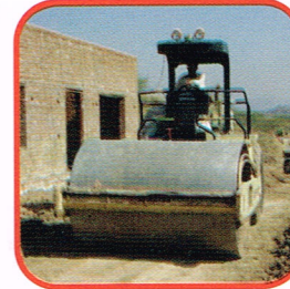
Workmen at KORT's New Complex
