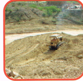
Ground Levelling at KORT's New Complex
