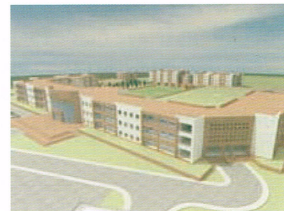
KORT complex in Jarrikas visualisation (above) and the construction so far (below)
