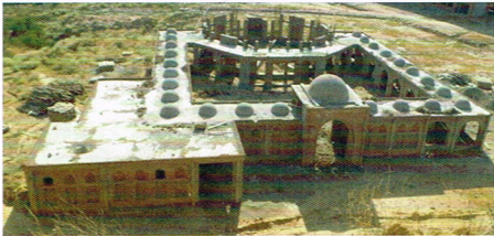
Masjid Under Construction
