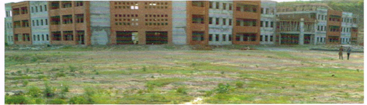
Three Floor School Building
